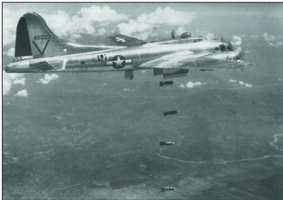
49th Squadron Pathfinder dropping bombs. Note radar dome below fuselage just aft of the wings. (Group Photo)
